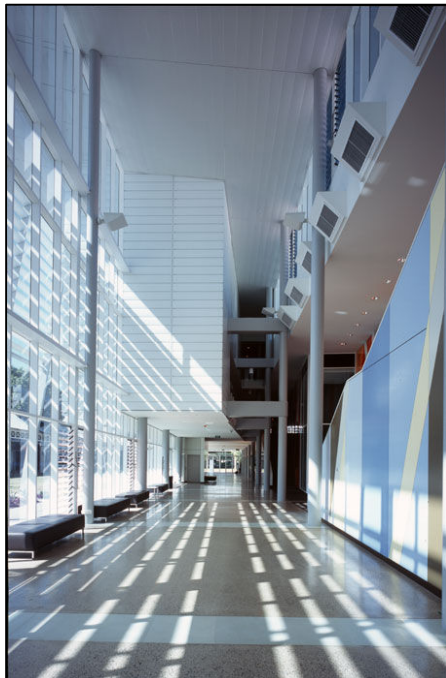
The Joan Sutherland Performing Arts Centre project incorporates Breezway Altair ™ Louvre Windows into this project to improve energy efficiency.
